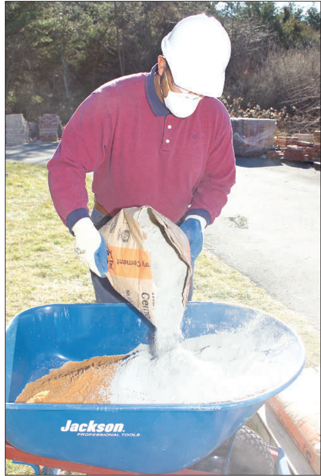
FIGURE 1-1 This construction laborer is a mason's tender.
